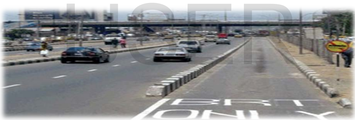
Figure 6: BRT Lane in Nigeria. (SOURCE: LAMATA .jpg)
